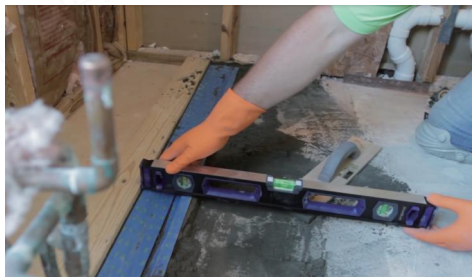
Step 10 Level the drain
