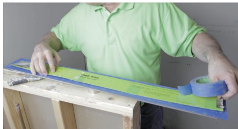
Step 10 Level the drain
