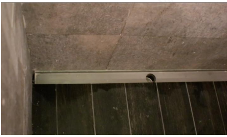
Step 16 Grout the tile
