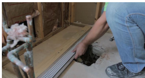
Step 7 Protect drain body and flange
