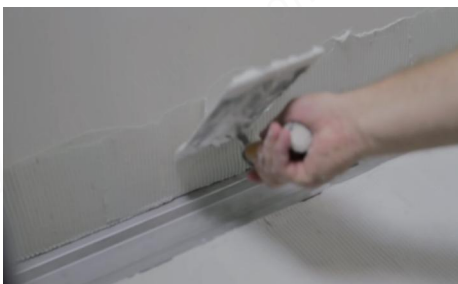
Step 16 Grout the tile
