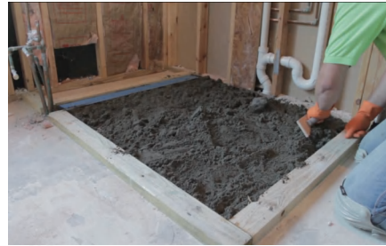
Step 12 Build a mortar perimeter guide
