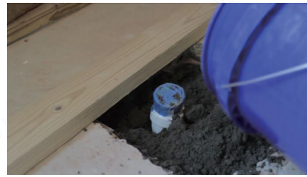
Step 9 Install and connect drain body
