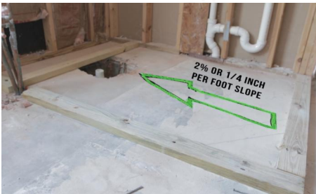
Step 11 Establish Mortar bed grade height
