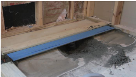
Step 11 Establish Mortar bed grade height
