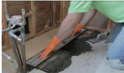
Step 12 Build a mortar perimeter guide
