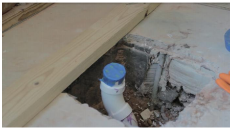
Step 8 Build the drain body support
