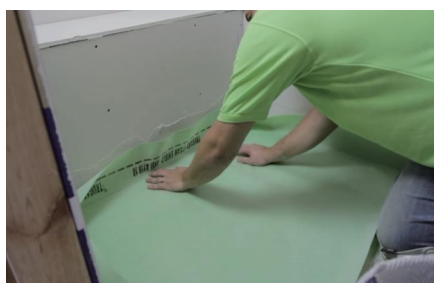
14.2 Apply sealant to drain flange 14.3 Place&embed membrane
